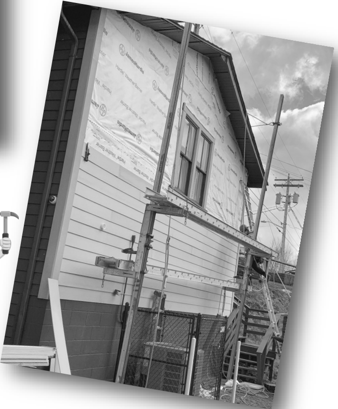
New Siding Going Up
