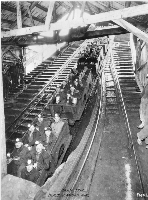
Mine 11's double track slope near the surface as a crew of miners prepared to descend underground.
